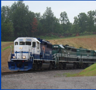
Railway Spur for Coal Mine, McHenry, Kentucky
