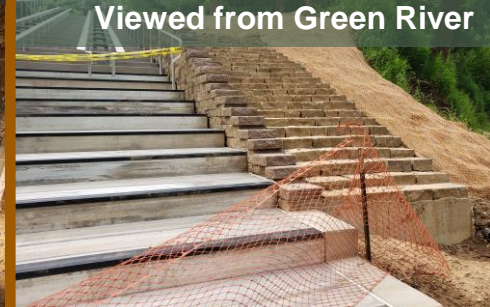
Post-Construction Launch Viewed from Green River
