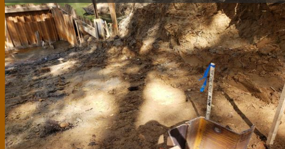
During Construction Staking
